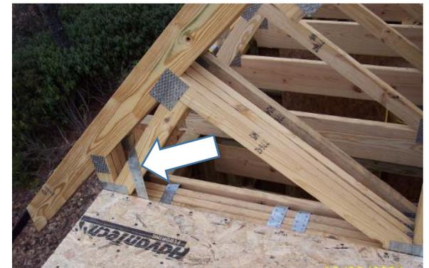
Typical attic truss strapping in a HOME ARCHITECTS® project.
